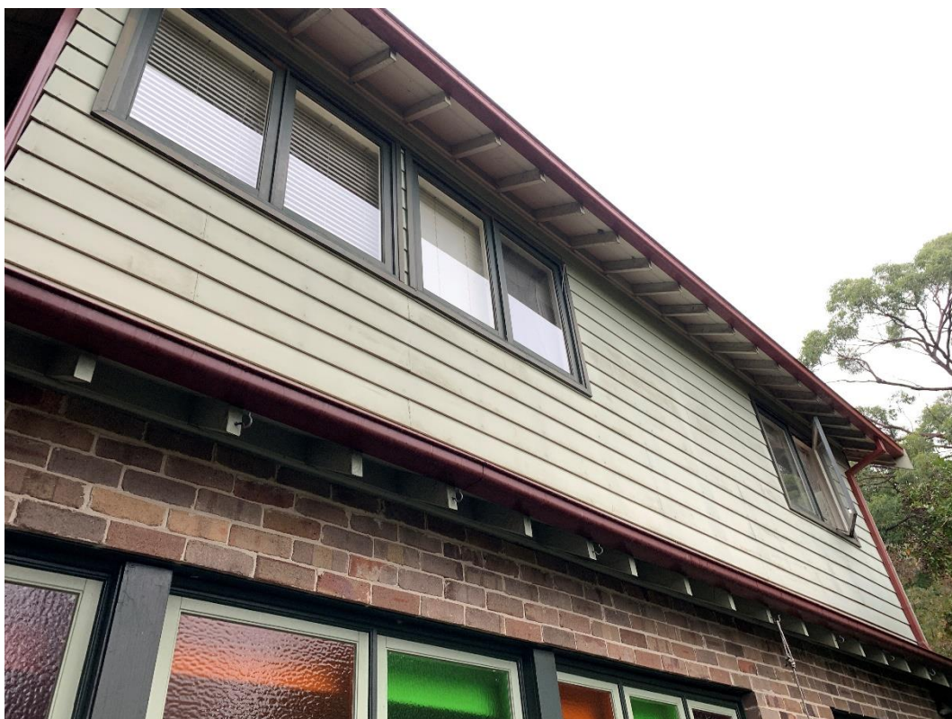
Photo 3: Showing second floor exterior wall panelling of 12 Marshall Avenue, does not contain ACM.
