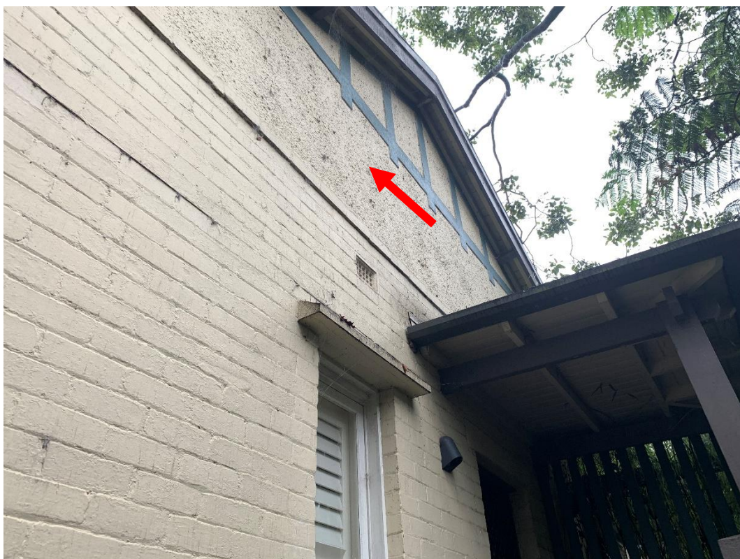
Photo 15: Showing exterior northern Gable of 3 Holdsworth Avenue, contains ACM.
