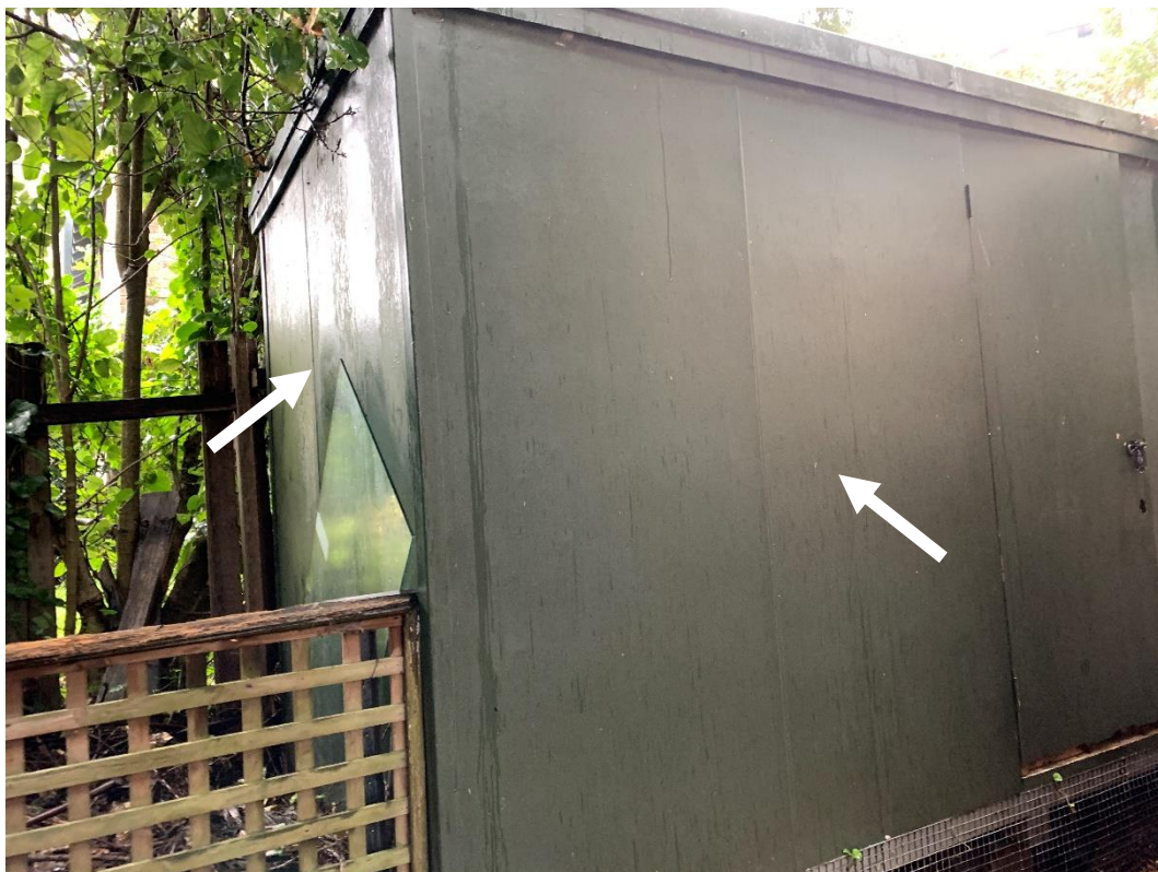
Photo 4: Showing exterior fibre-cement walls of side sunroom at 12 Marshall Avenue, contains ACM.
