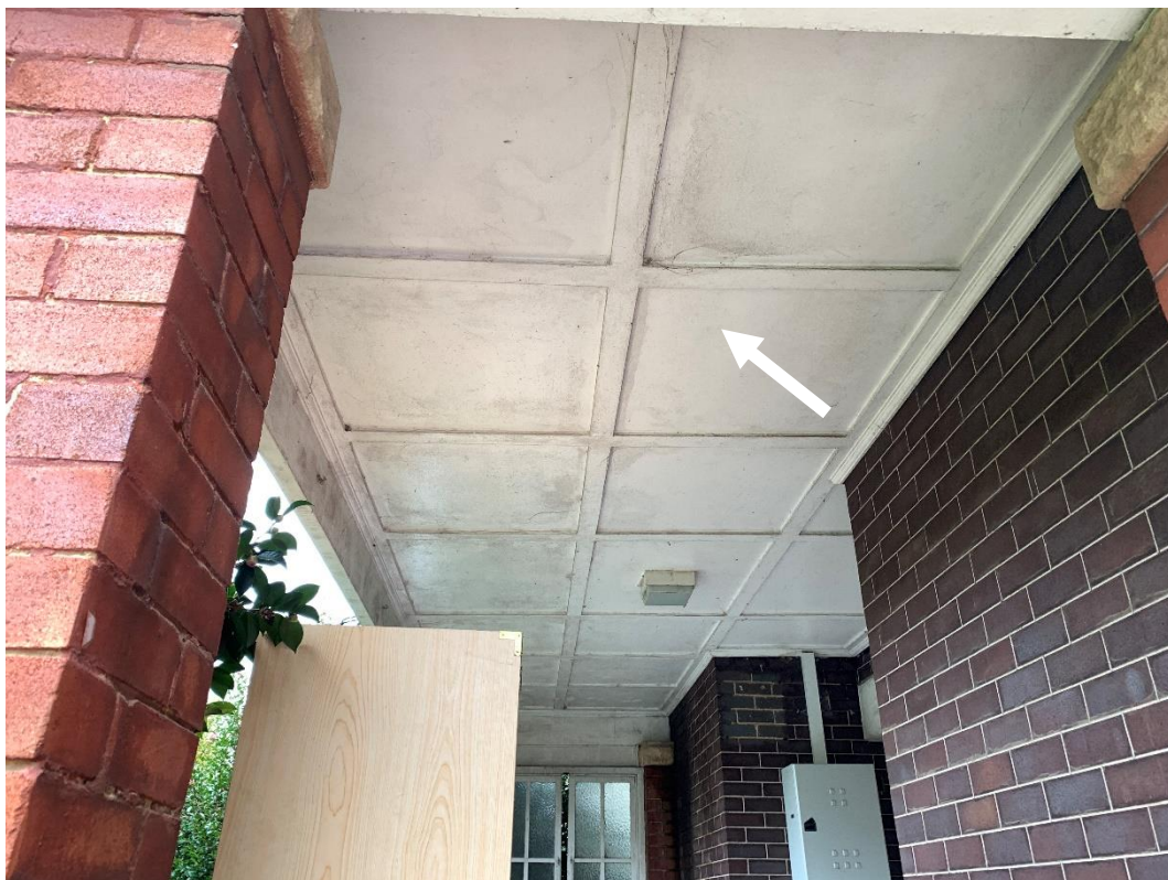
Photo 6: Showing front verandah ceiling of 10 Marshall Avenue, contains ACM.
