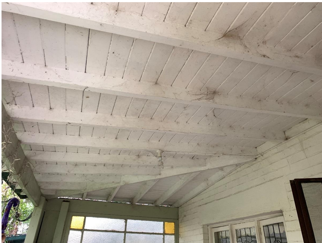
Photo 10: Showing exterior eaves of 1 Holdsworth Avenue, does not contain ACM.
