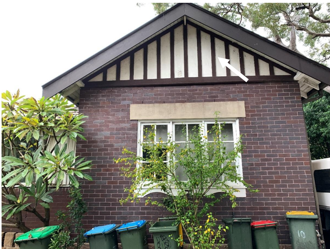
Photo 5: Showing northern gable of 10 Marshall Avenue, contains ACM.
