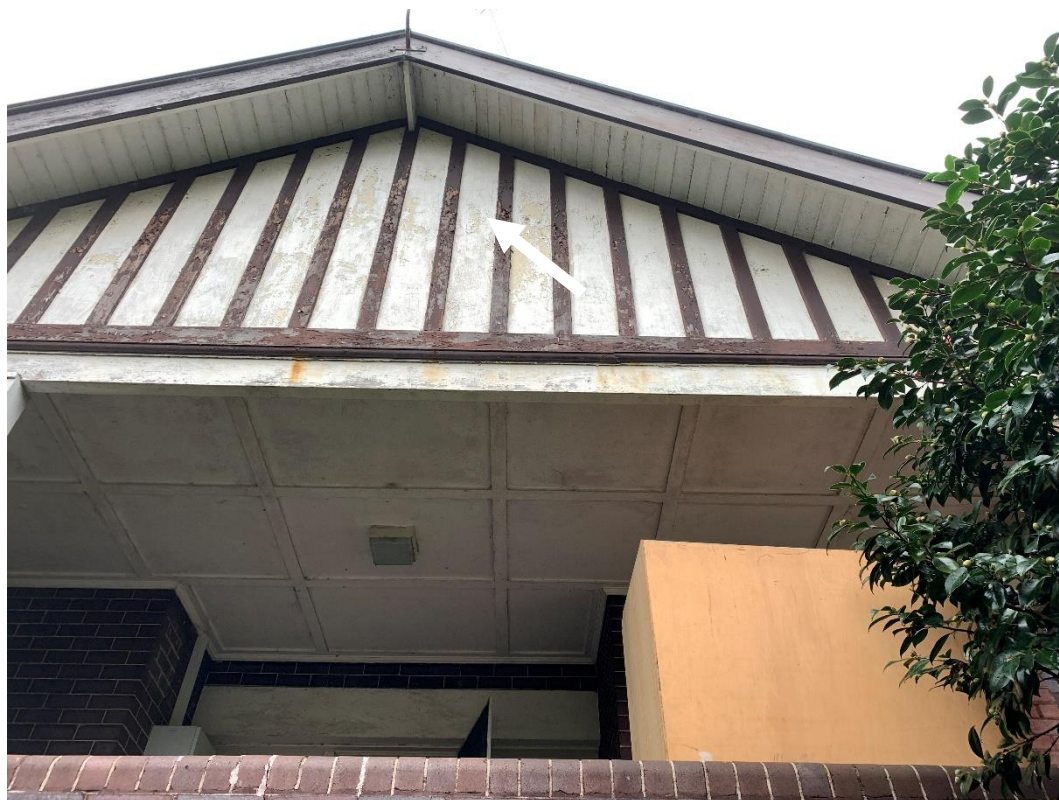
Photo 8: Showing eastern gable of 10 Marshall Avenue, contains ACM.
