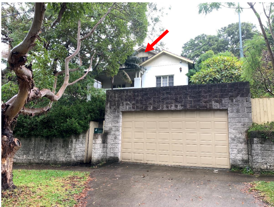
Photo 9: Showing eastern gable of 1 Holdsworth Avenue, St Leonards, contains ACM.
